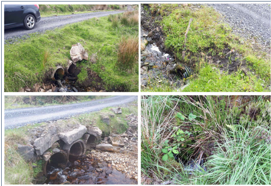
Photo 3: Examples of Pipe Culverts (Source, FT)
