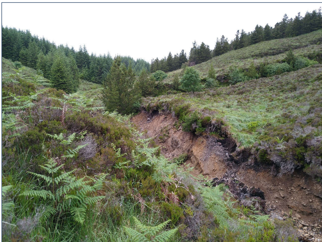
Photo 4: Eroded Streambanks and Exposed Subsoils
