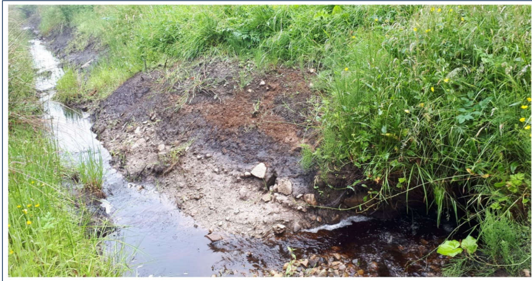
Photo 5: Drainage Ditch With Exposed Subsoil Beneath Peat (Source: FT)
