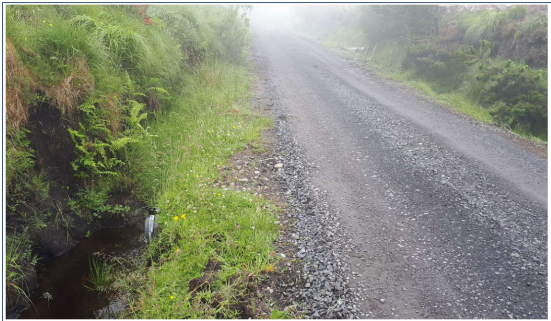
Photo 6: Crushed Aggregate Road, Pipe Culvert Across Road, and Drainage Ditches on Both Sides of Road
